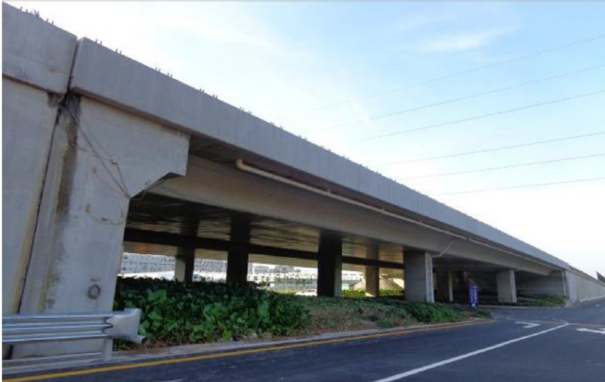
Maluanshan bridge (Shenzhen, L=3\times30 m): (a) overall view of IAB, (b) details of integral abutment and pile
