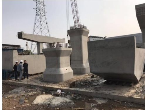
Precast Column and Cap Beam
