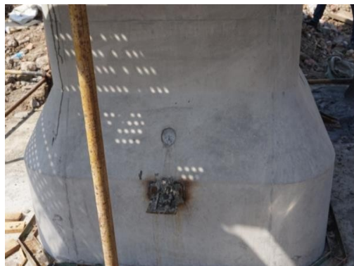
Grouting of Column- Pile Cap Joint Completed
