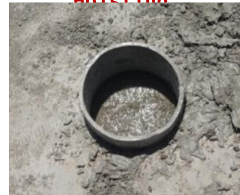
Grouting of Column-Cap Beam Joint Completed
