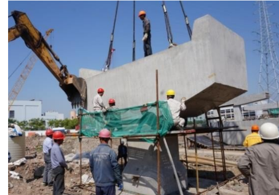
Precast Cap Beam Hoisting
