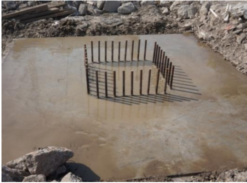
Pile Cap and Rebar Arrangement
