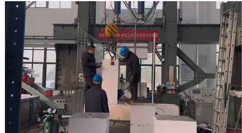
Assembling process of specimen SCDP-BRBs
