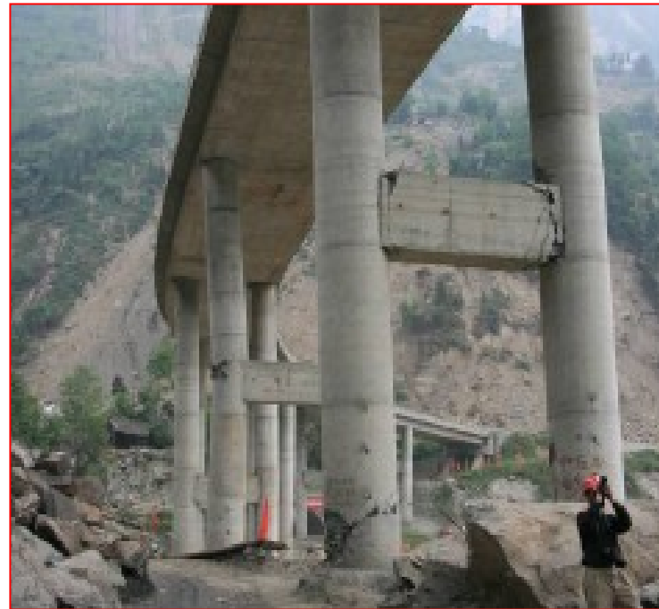
Typical earthquake damage of double-column piers
