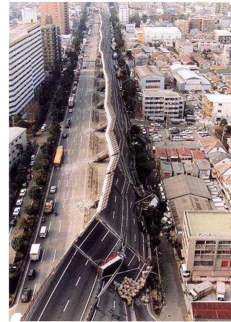
Piltz type elevated-girder bridge(RC structure)
