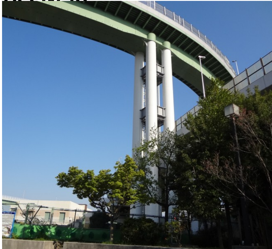
Ebie JCT 2012(1 pier) , Osaka, Japan
