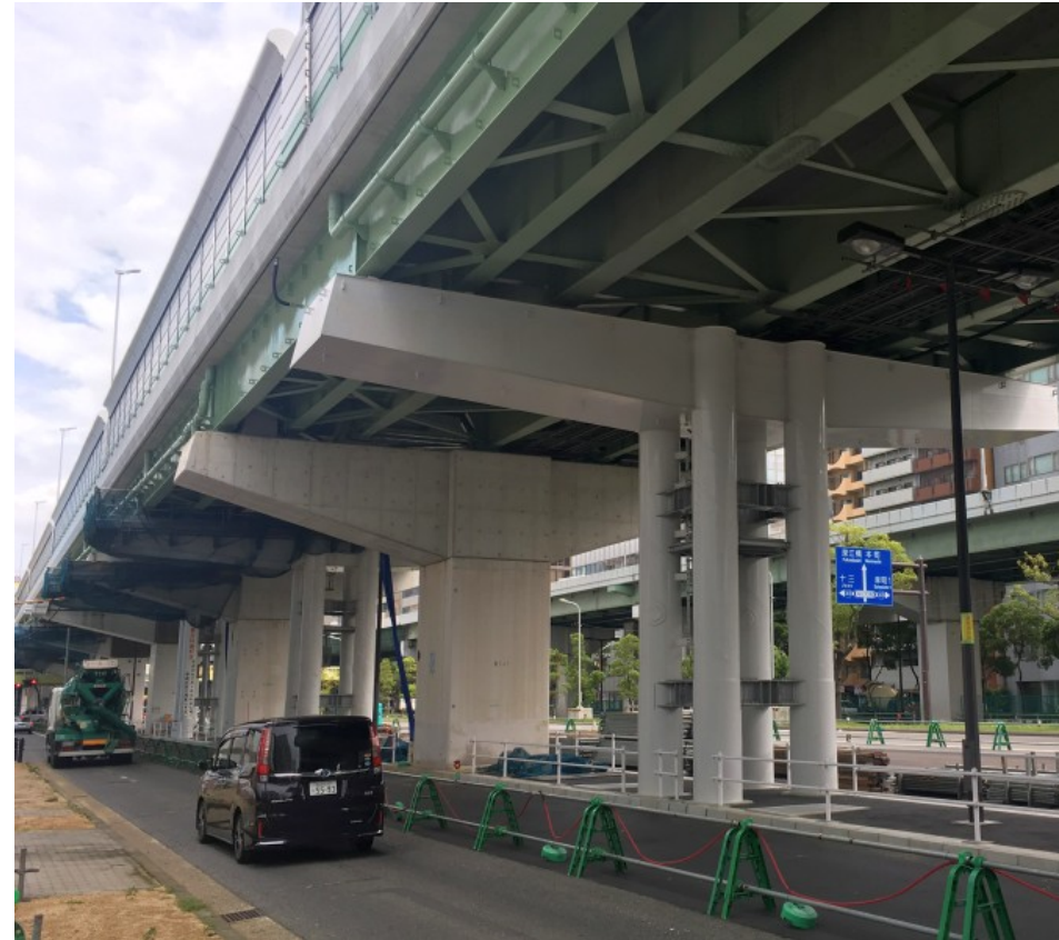
Nishisenba JCT ( 12 piers ) 2018, Osaka, Japan
