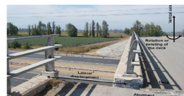
Torsional response, 2010 Chile earthquake
