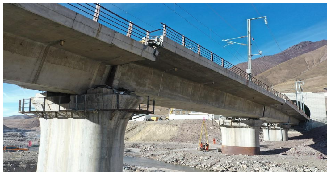
Seismic Damage of High-Speed Railway Bridges
