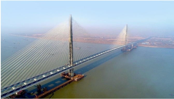
Wuhu Yangtze River Second Highway Bridge
