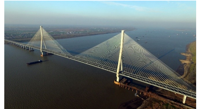
Wangdong Yangtze River Highway Bridge
