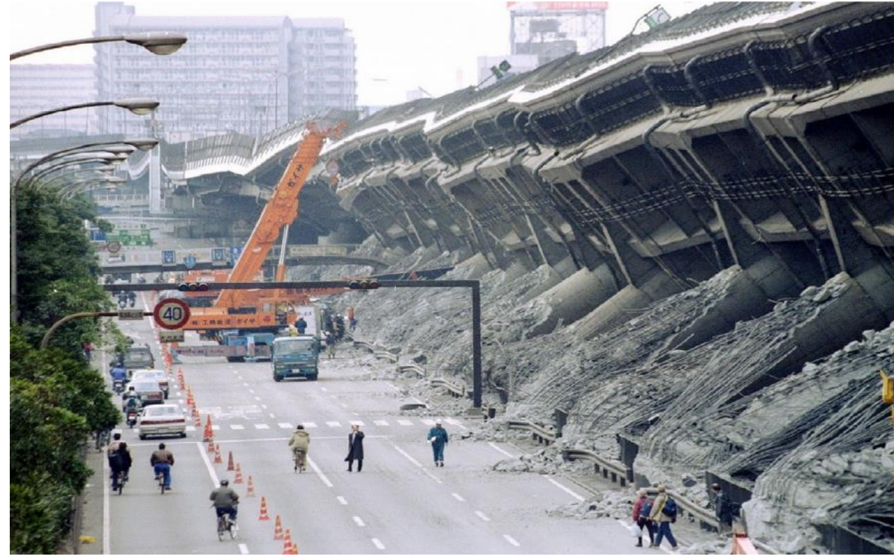
Difficulty in demolition and reconstruction
